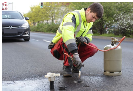
Installation of wireless sensor nodes in the road surface as part of the sMobility field test in Erfurt. Photograph: IMMS.
