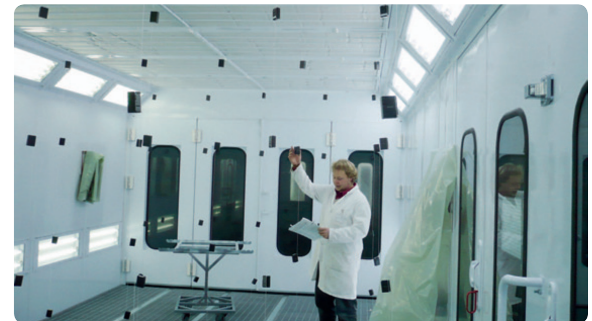
Analysis of production conditions inside a spray booth with wireless sensor networks. Source: IMMS
